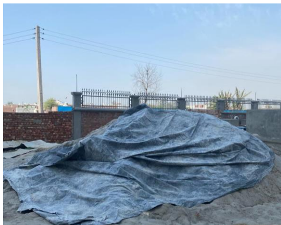
Construction material is covered with sheets
