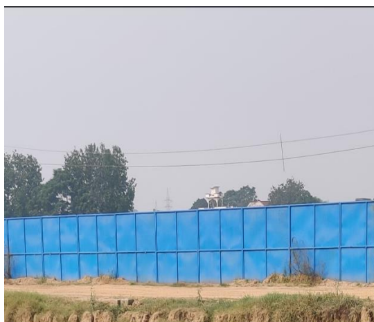
Sheets installed on site boundary as wind breaker
